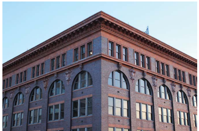
The 116 year-old Textile Building in downtown Cincinnati was transformed from office space to residential units.
