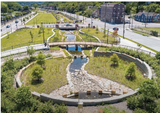
The Lick Run Greenway, completed in 2021 by Greater Cincinnati Metropolitan Sewer District, is an example of a large-scale green infrastructure project that reduces combined sewer overflows. Photo courtesy of MSD.
