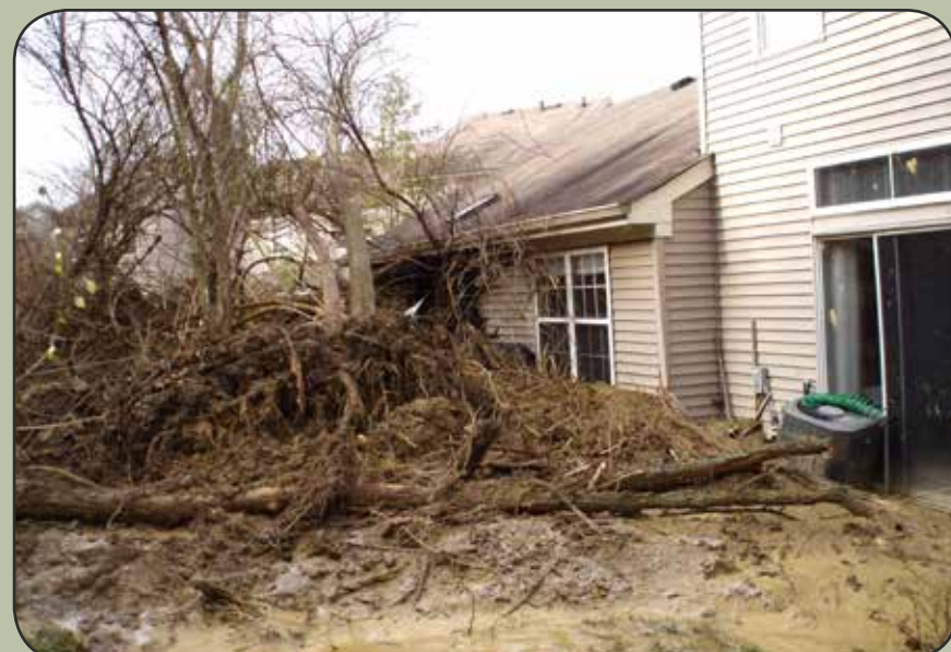
Figure 9. Jumbled trees and mud at the toe of a translational slide that damaged a condominium in Bellevue, Kentucky. Landslides can damage property at the top or bottom of a hill.
