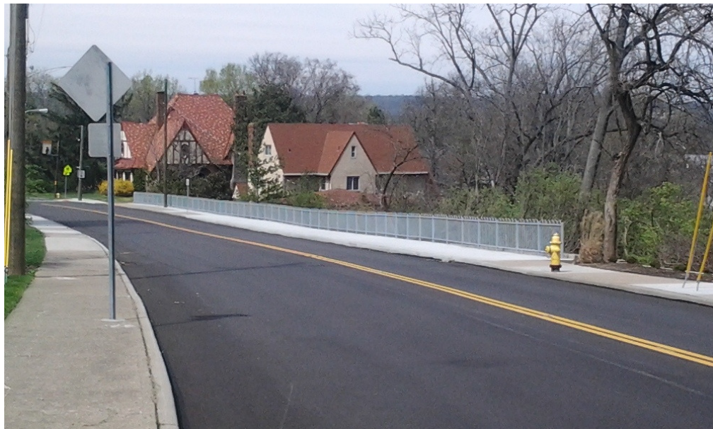
Clinton Springs looking west after repairs.
