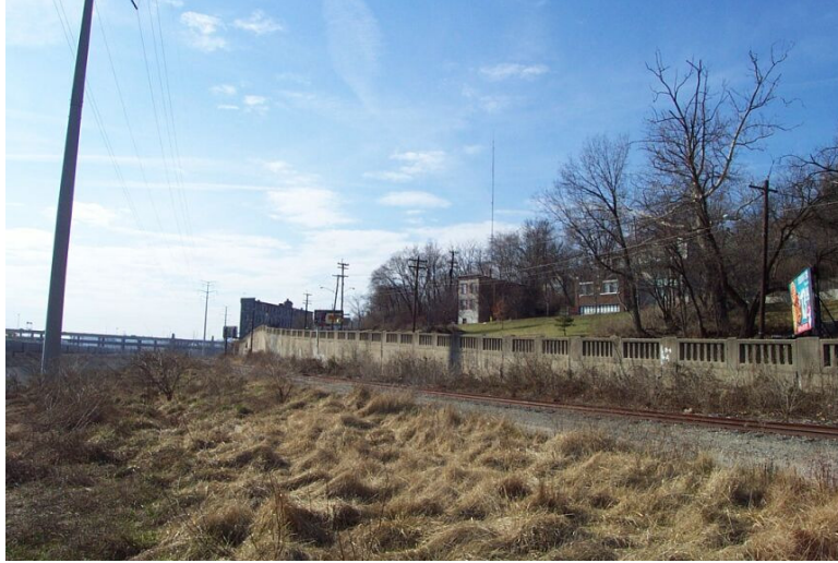
Southern portion of Cummins Street retaining wall from below.
