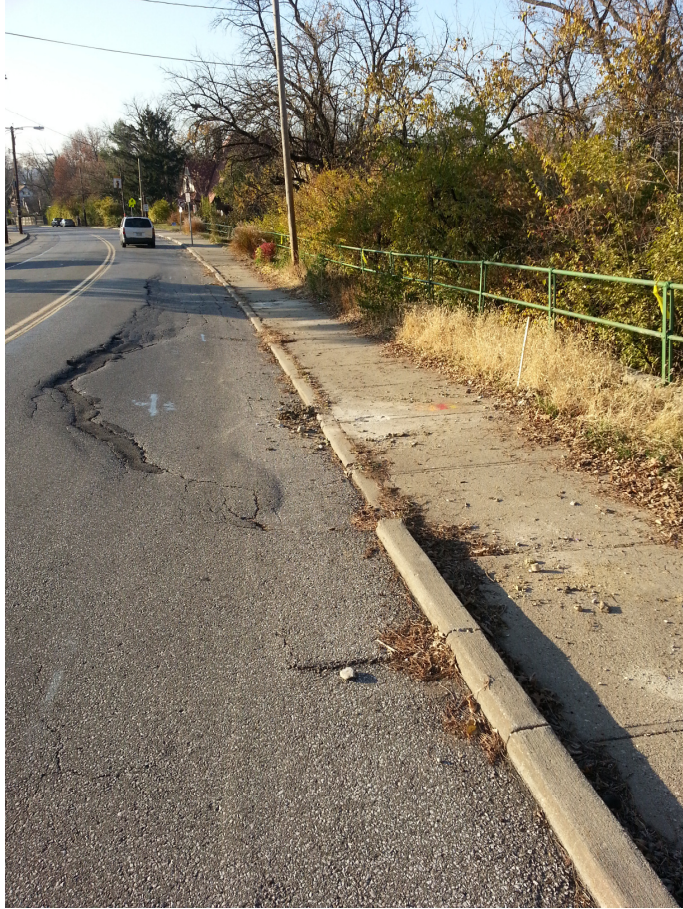
Clinton Springs looking west prior to repairs.
