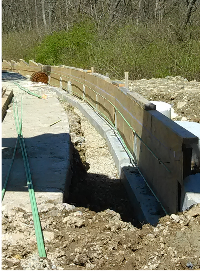
Forming for wall cap on Ridgetop Way Pier Wall Extension.
