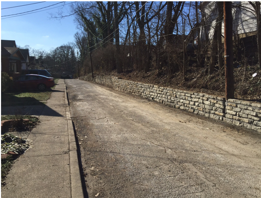
Hoadly Court looking south after wall repairs.
