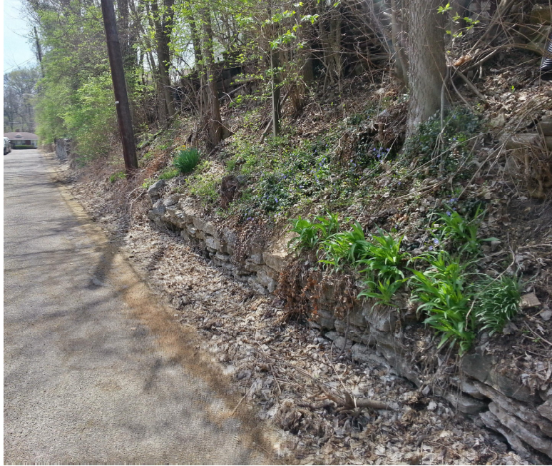
Hoadly Court looking south prior to wall repairs.
