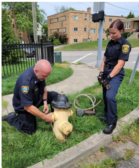
Exhibit 3: CFD Firefighters servicing a fire hydrant in Hyde Park.
