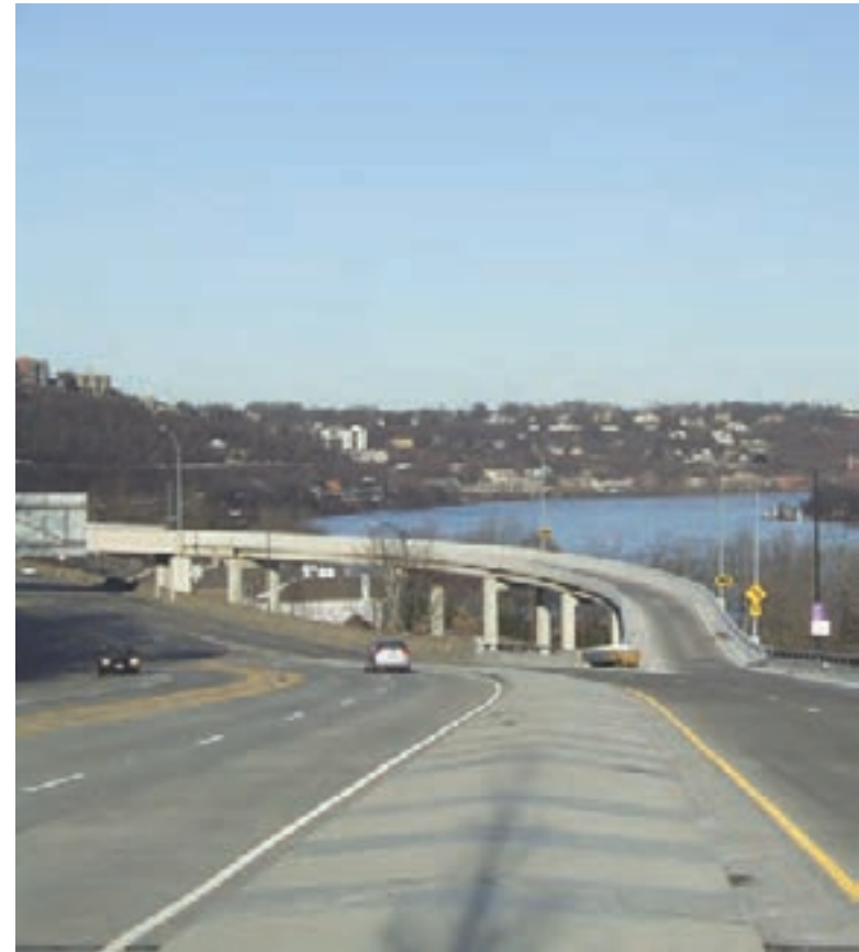
Columbia Parkway from the 5th Street Viaduct at Martin Drive
