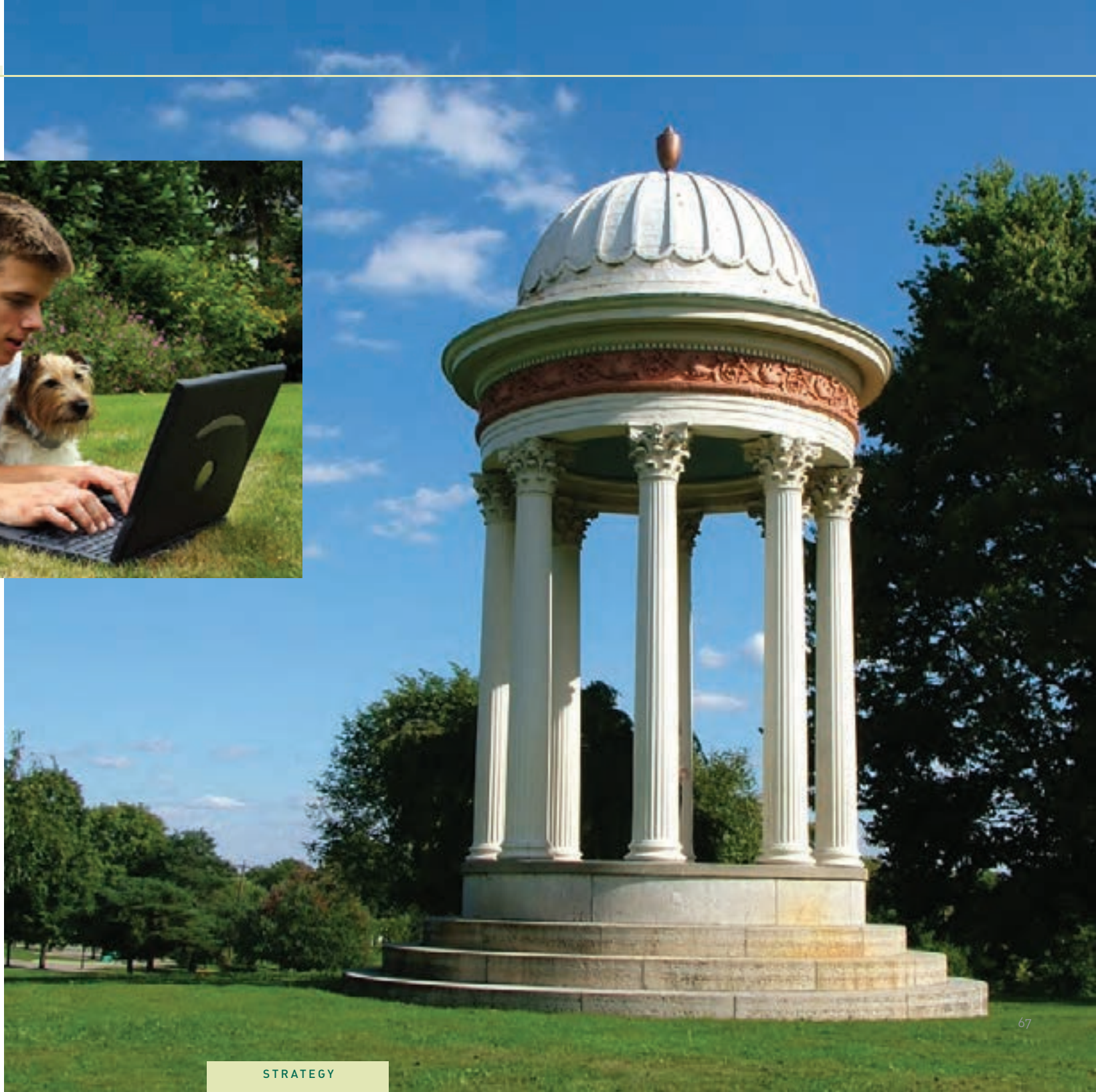
Located on the east lawn of Mt. Storm is The Temple of Love, a structure dating to c.1850.
